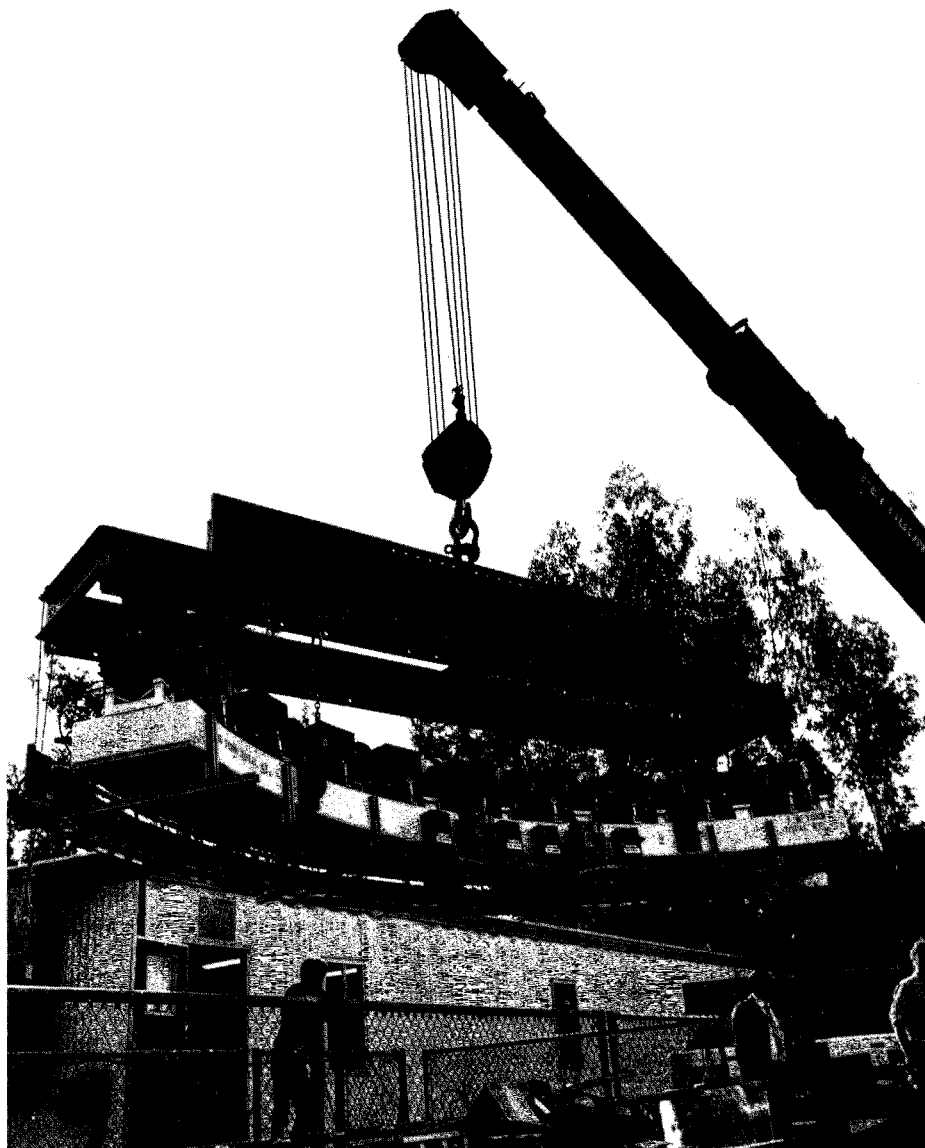
Construction work for the damping ring for the proposed SLC linear collider at SLAC has been proceeding even with the main linac in operation. Here a raft of magnets is seen being lowered into the damping ring vault. Beam has been carried through the linac-to-ring transport system. (Photo Joe Faust)
